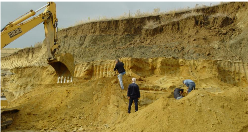
Figure 1: Start of the excavation, July 2007.
