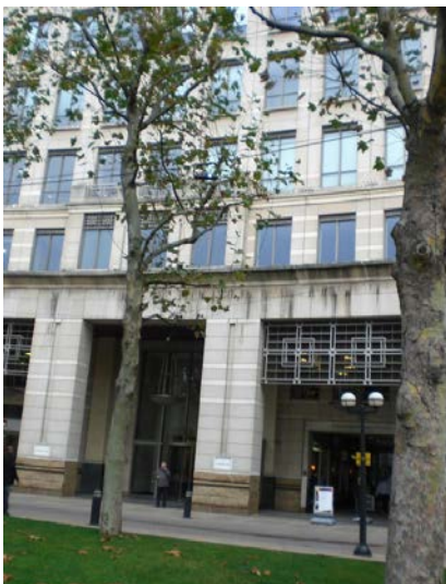
Figure 1. The main building of EMA in London 7 Westferry Circus.
